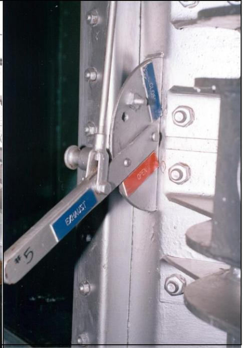
**Fig. 99:** Closeup of lever used to open and close exhaust stack.
