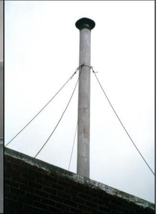
**Fig. 103:** Exhaust stack.
